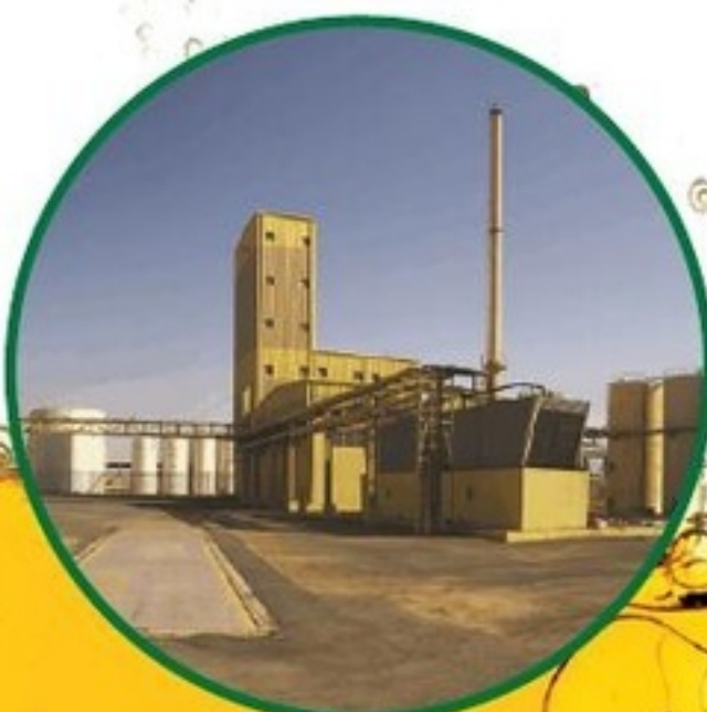
Used Engine Oil Re-Refining Plant
