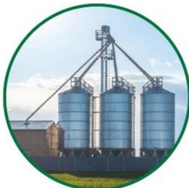
Silo and Seed Cleaning Plant
