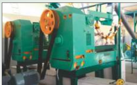
Installed in India
