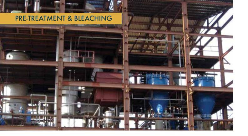
he process of removing visible impurities and colour pigments from vegetable oils is known as bleaching. Traces of gums, soaps are removed as an added advantage. This process is typical to both physical and chemical refining - the only difference is that crude oil is pre-treated in physical refining, whereas, in chemical refining, neutralized oil can be directly fed into the bleacher.
