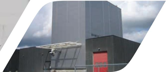
Cimbria square silos are manufactured to store many different smaller quantities of grain products, with capacities of up to 20,000 m<sup>3</sup> or even higher. Built with heavy, trapezoidal, or face-plated steel plate, and with cell sizes up to 4m x 4m, they can be delivered in several combinations. Each silo is individually and precisely designed to meet the customer's specific demands.
