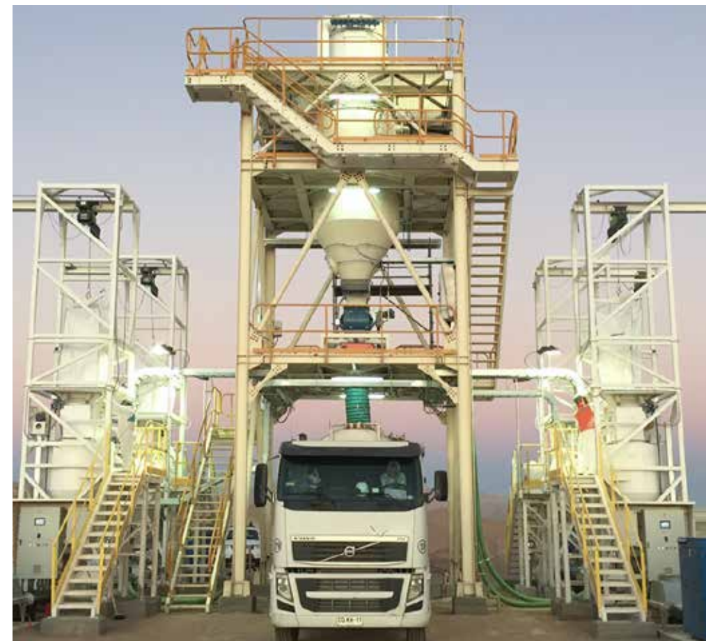
Complete Logistic Centre
