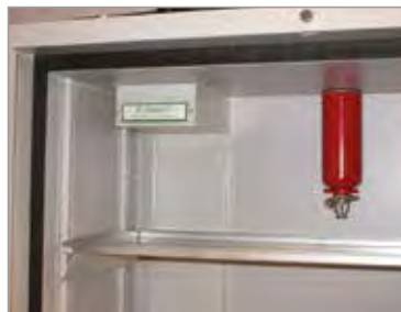
Fire-extinguisher installed in a safety cabinet
