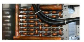
Continuous research for energy-saving solutions is the basis for the technology of the condenser and heat recovery unit with 8-litre exchange coil, which can be installed on the entire LCF series, to supply the machine with cold water.
