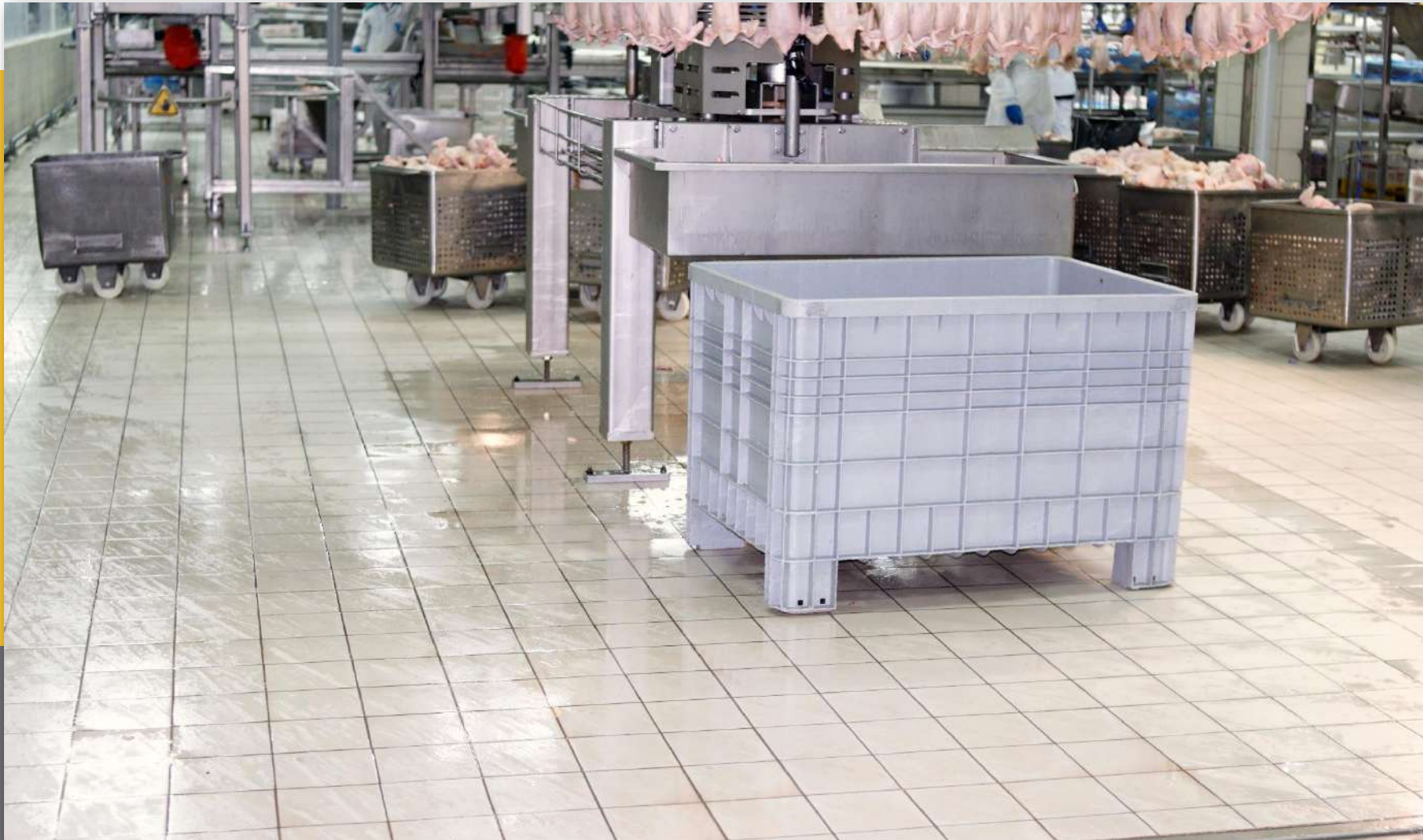
EFD System application with Vibration Tiling System.
