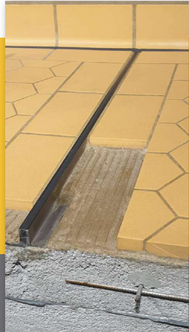
St. Steel L-Profile Expansion Joint X-Section
